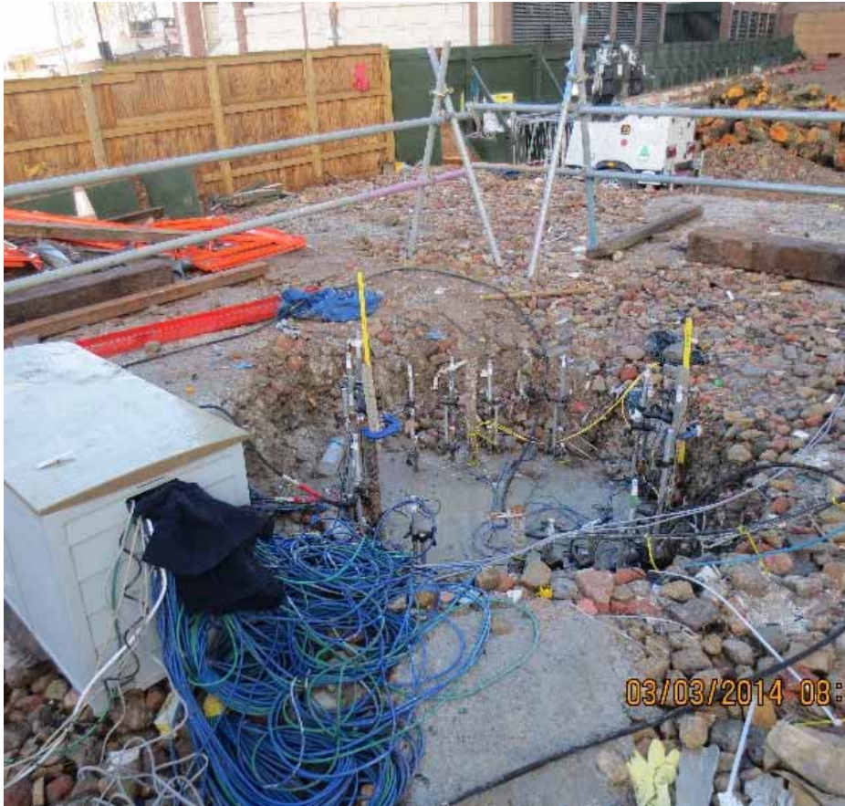
Conventional Strain Gauge System
